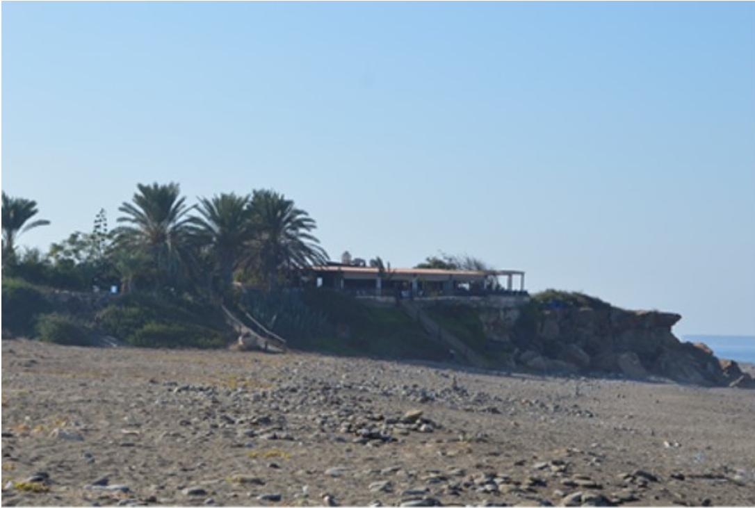
Illegal restaurant at South Lara
