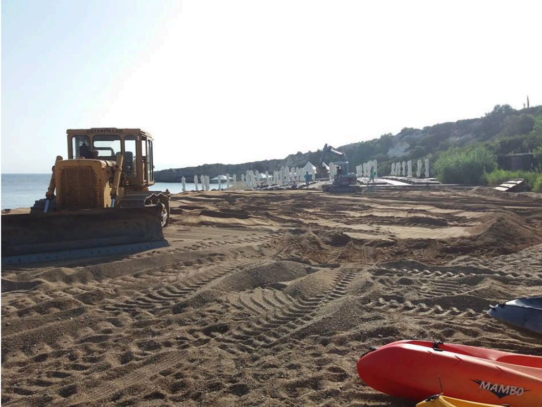
Illegal beach intervention at Asprokremmos
