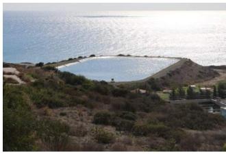
Tertiary treated water tank (Moni Wastewater treatment plant – LIM021)
